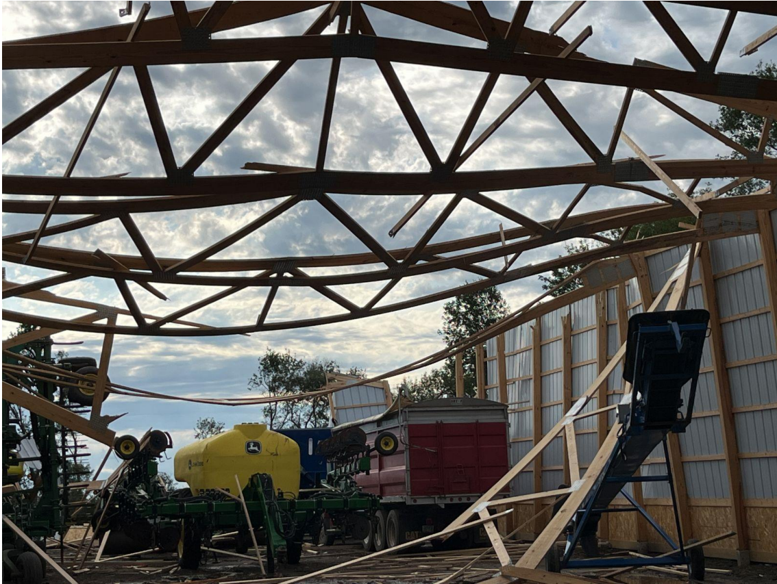
Damage to a Farm Building North of Courtenay. (NWS Bismarck Damage Survey)
