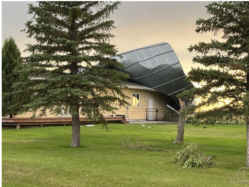
Thunderstorm damage near Pettibone, North Dakota. Large Grain Bin was Dislodged from its Foundation and Rolled to the West, Wrapping Around the Side of a House. Photo and Summary from NWS Bismarck damage survey.
